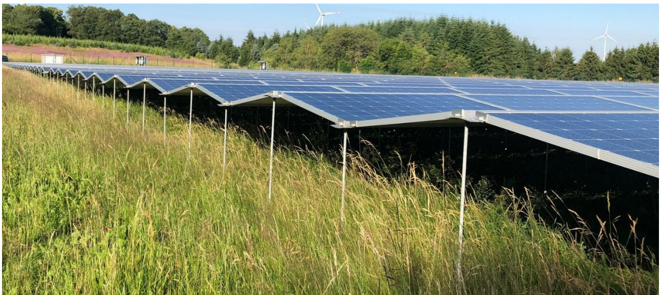
Figure 1: East-West mounted solar system
