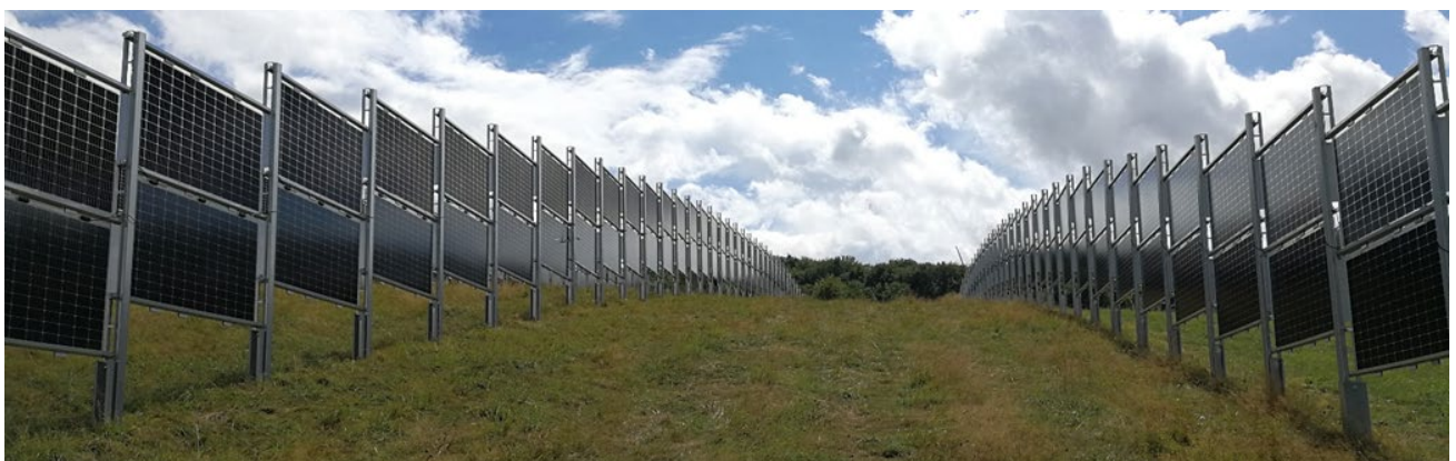
Figure 4: Vertically mounted bifacial modules (source: Next2Sun)
